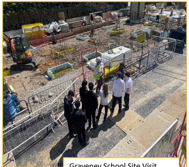
Graveney School Site Visit
