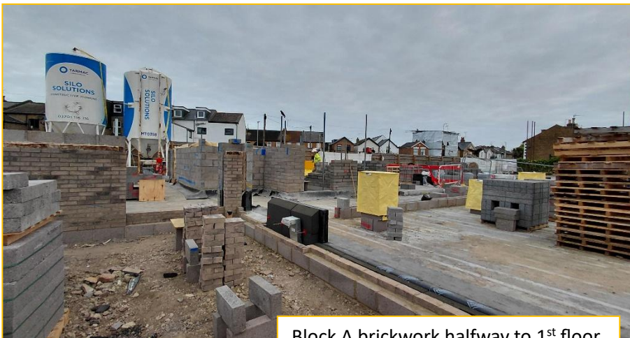
Block A brickwork halfway to 1 st floor
